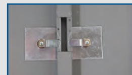
User doors reinforced at latches
